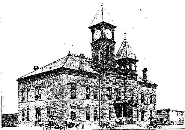
COVINGTON COUNTY COURT HOUSE.
